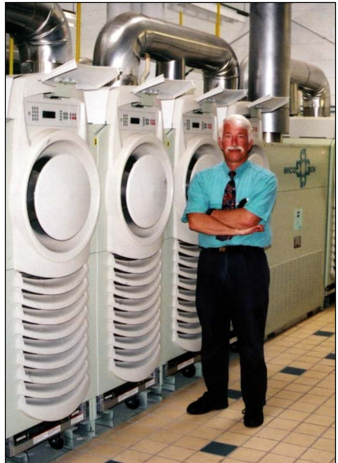
Robert Bechtold, the owner and president of Harbec Plastics Inc., displays several of the state-of-the-art Capstone microturbine generators used to power his company. Photo by Patrick O'Mahen
