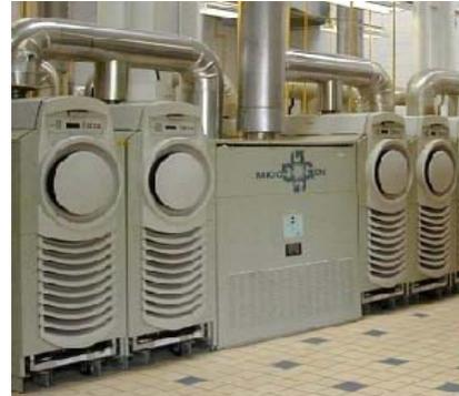
**Four Capstone micro-turbines coupled with a heat exchanger at Harbec.**
