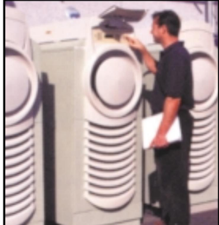
**HARBEC CEO BOB BECHTOLD** installed 20 micro turbines to supply his Upstate company with power. It is the largest micro-turbine installation in the world. Technician pictured above monitors one of several micro turbines.
