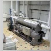
Use of exhaust heat for absorption A/C means reduction of moisture in plant air which reduces the need for use of electric material dryers by as much as 75%.
