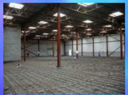
17,000' of 1" Diameter tubing for radiant floor heating
