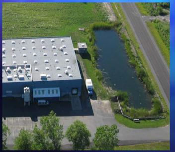
850,000 gallon pond to provide water capacity sufficient for sprinkler system and to provide cooling and make-up water to compliment process water loop thanks to help from NY ESD
