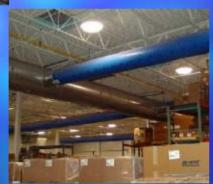
Air-to-water heat exchanger delivers hot and cold water to the rest of the building's HVAC system and uses high efficiency Air Sox to deliver conditioned air.
